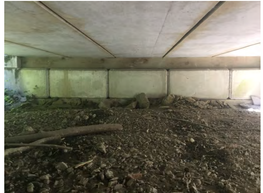
Left Bank Abutment when facing downstream
