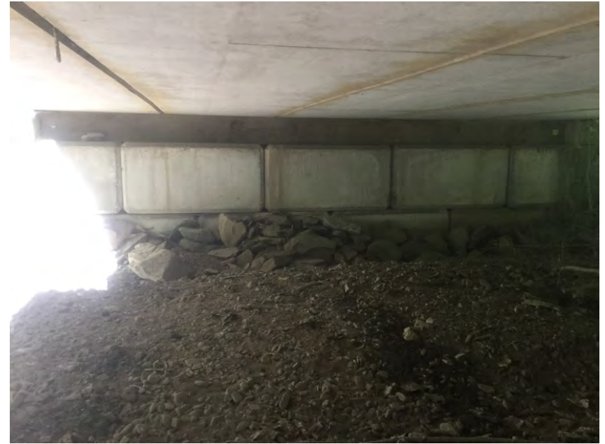
Right Bank Abutment when facing downstream
